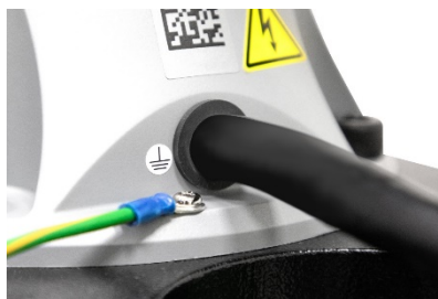
Figure 24: Securing the ground wire with the robot
